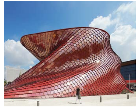
Vanke Pavilion (EXPO 2015), Mailand, IT © Hutton + Crow, Studio Libeskind
